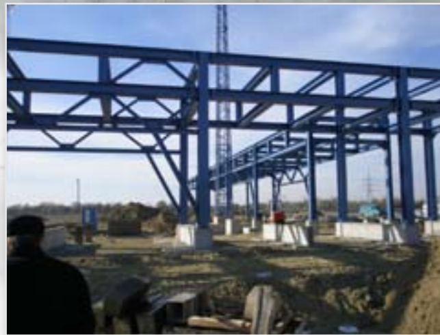
One section of the pipe bridges
