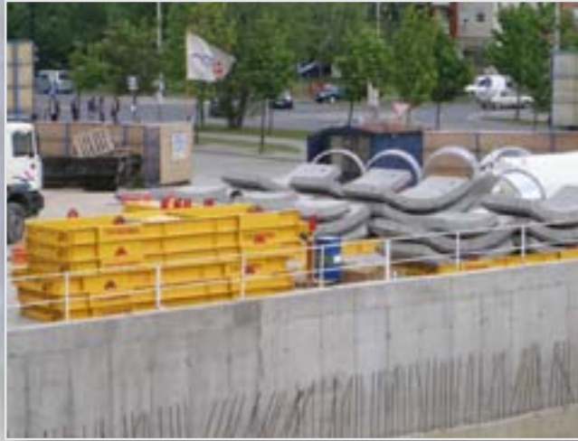
The lifting frames (some loaded)
