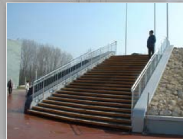
Laminated wood stair construction
