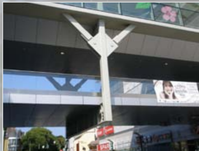
Part of steel bridge
