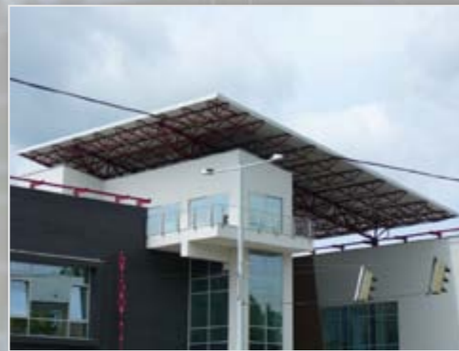
Foreroof of main entrance
