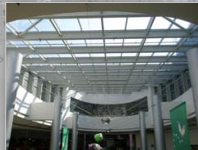
Steel construction of one of the elliptical glassholder
