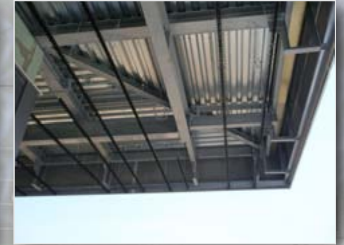
Hot dip galvanized steel cosntruction
