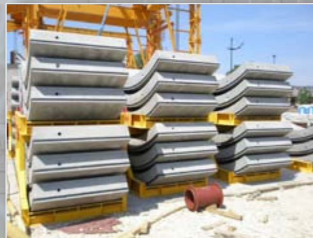
Frames loaded with concrete segments
