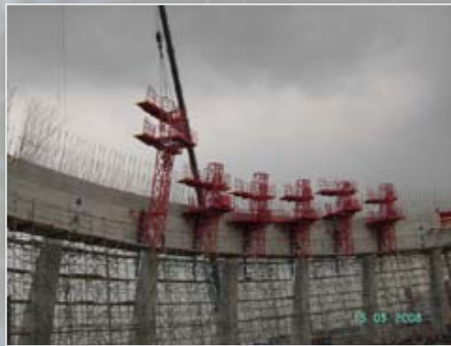
Pre-assembling the lifting steel towers, platforms
