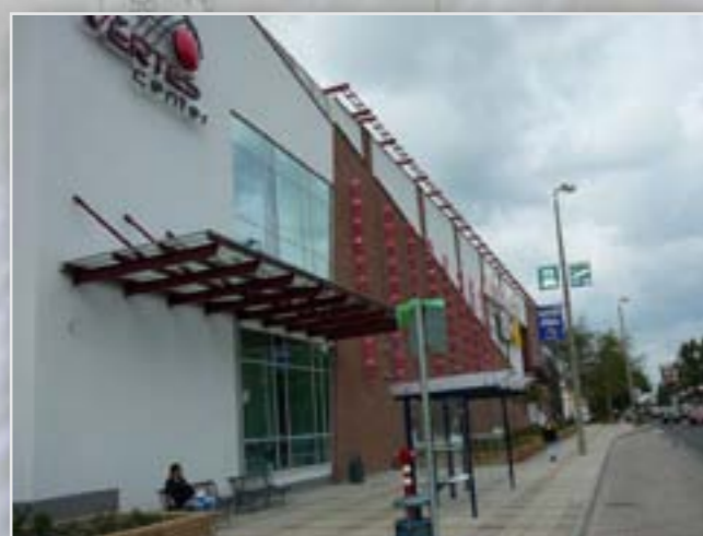
Glass foreroof on facade
