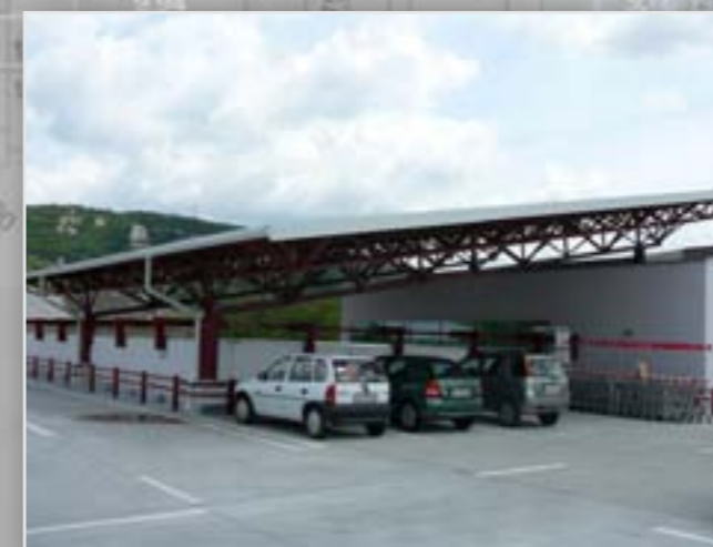
Foreroof of main entrance from side
