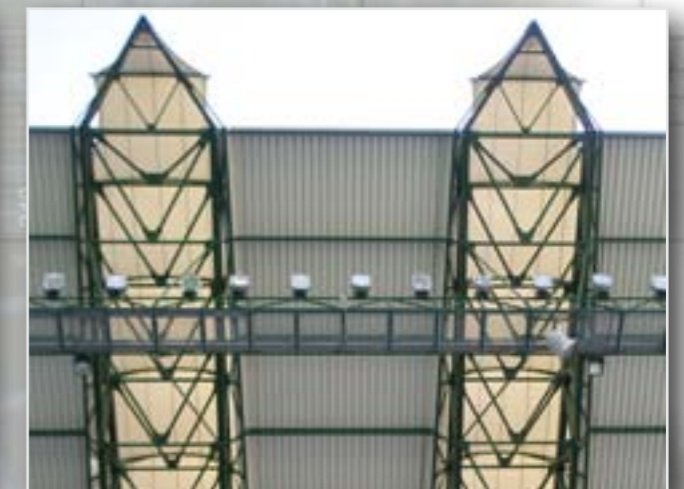
Huge truss-beams holding the roof
