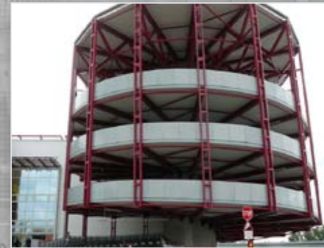
Spiral car ramp from side
