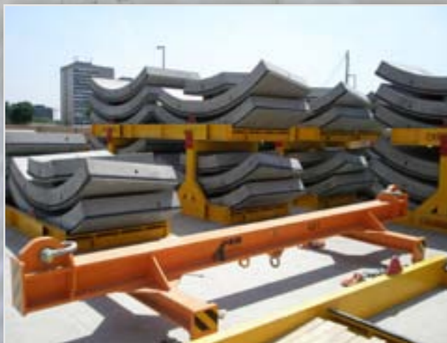
Frames loaded with concrete segments
