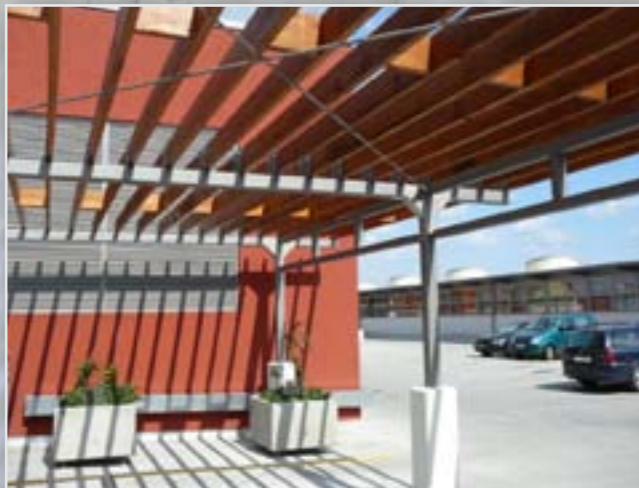
Steel and wood combined pergola
