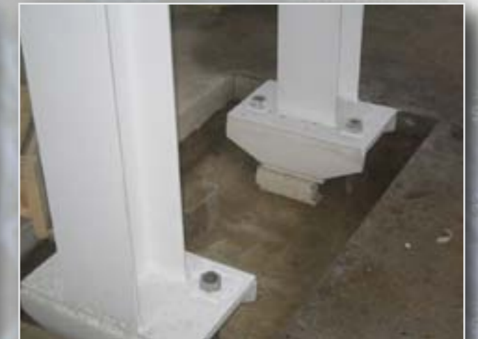
Fixing of columns with concreting
