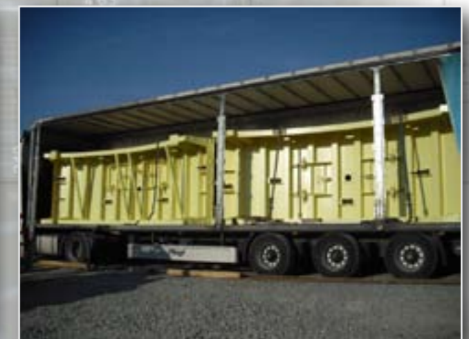
Formwork panels arriving from Hungary
