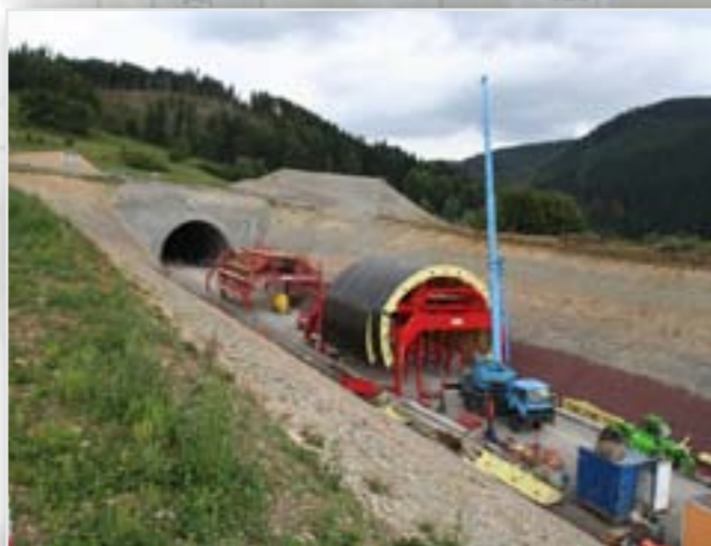
One set of formwork car is almost ready
