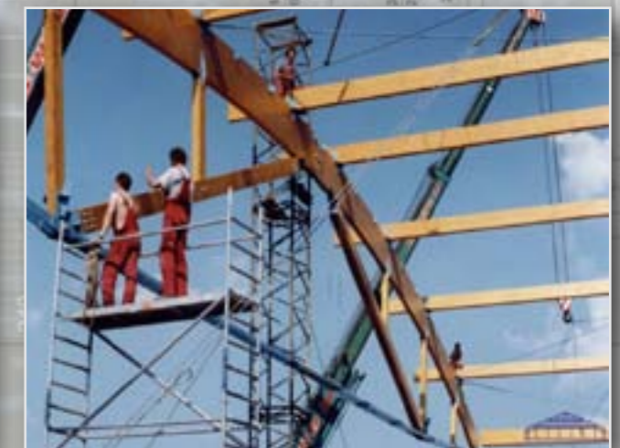
Installation of the wooden roof structure
