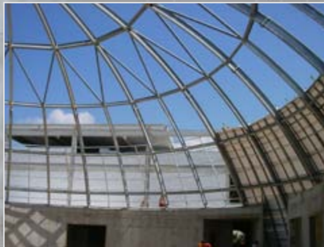
Steel construction from inside
