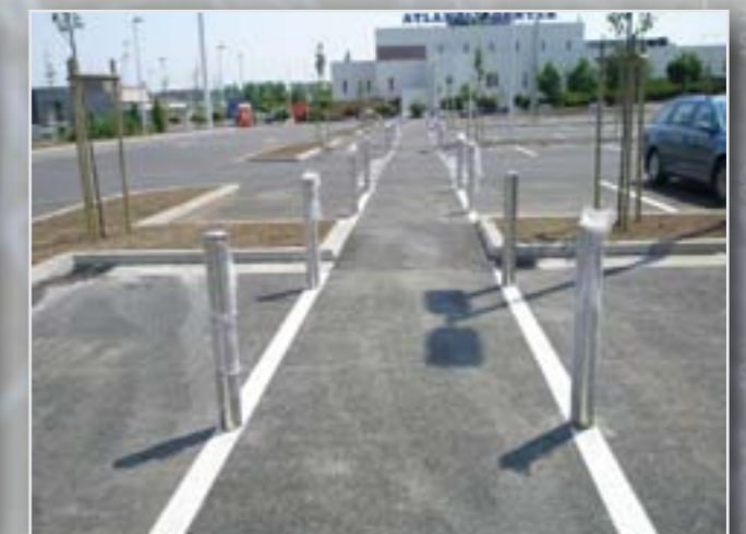
Stainless steel protective columns
