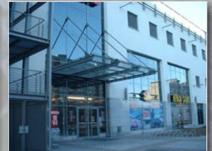
Glass covered steel foreroof
