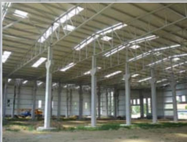
Concrete columns with steel truss-beams
