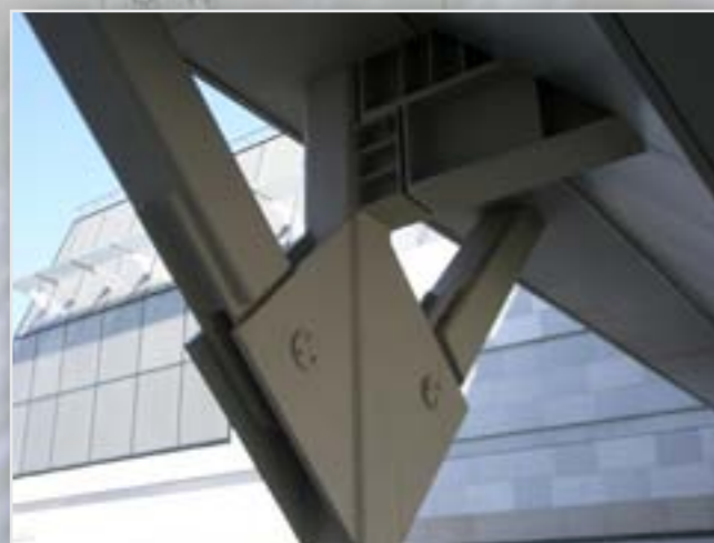
Steel part of bridge construction
