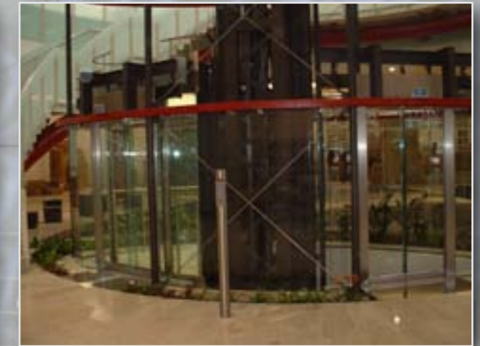
Panoramic elevator - Protection against reaching-in
