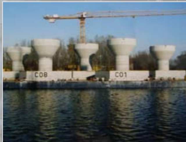
Fixing of columns with concreting
