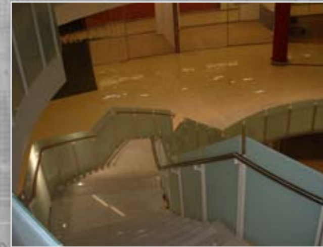
Railing of panoramic stair
