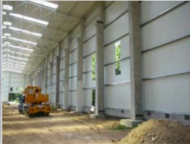
Truss-beams and purlins of "Skoda" hall
