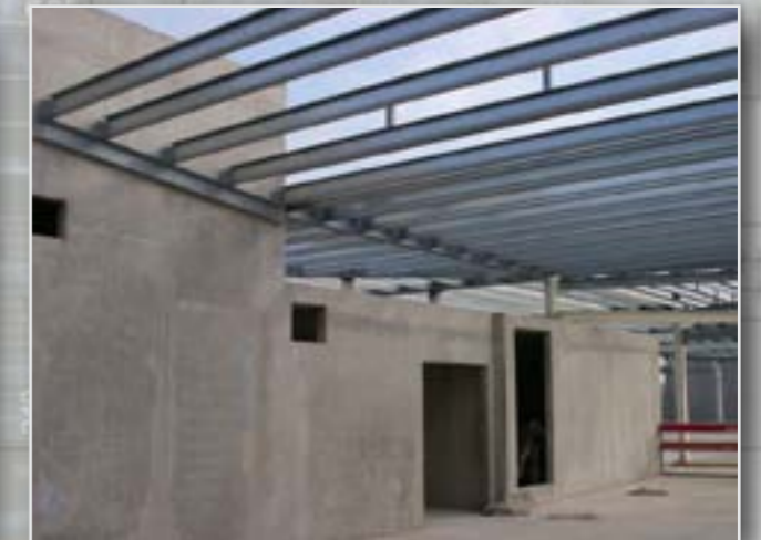
Connection of concrete wall and purlins
