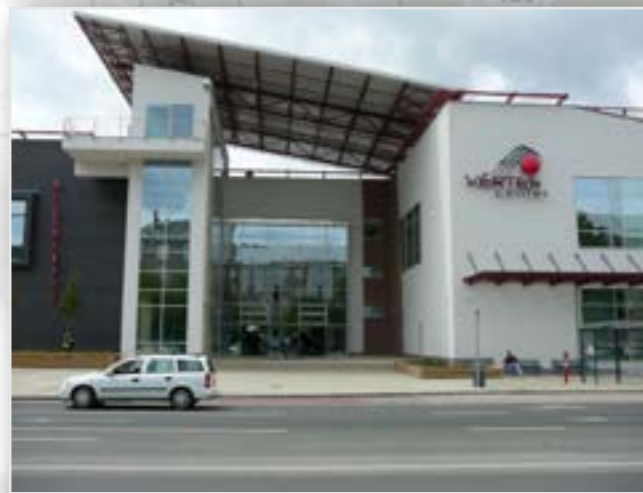
Wide span foreroof of main entrance
