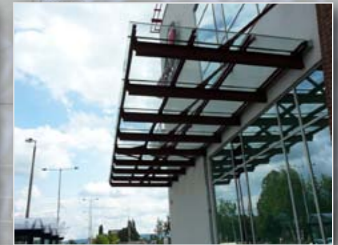
Glass foreroof on facade
