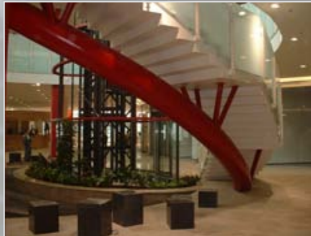
Steel tube construction of panoramic stair
