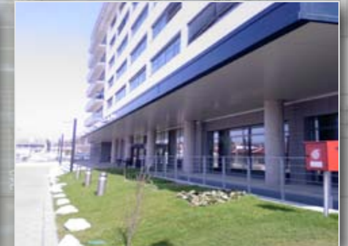
Main foreroof and covering
