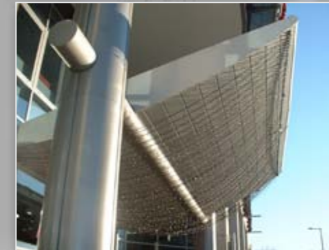
“banana” foreroof of main entrance
