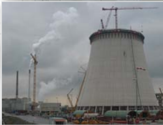
Concrete tower building in progress
