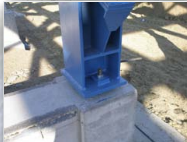
Column fixing detail
