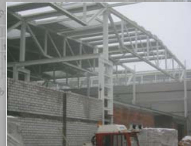
Endwall of the hall
