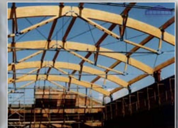
Installation of the wooden roof structure
