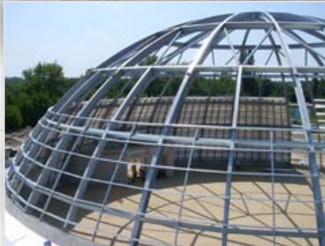
Sphere steel construction
