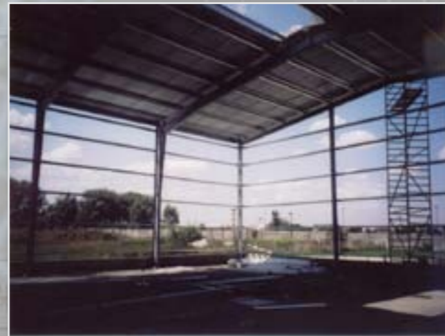
The hall under construction
