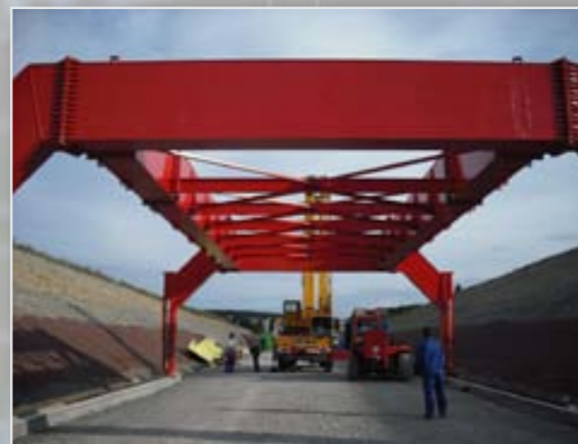
Base construction with welded square-tube profiles
