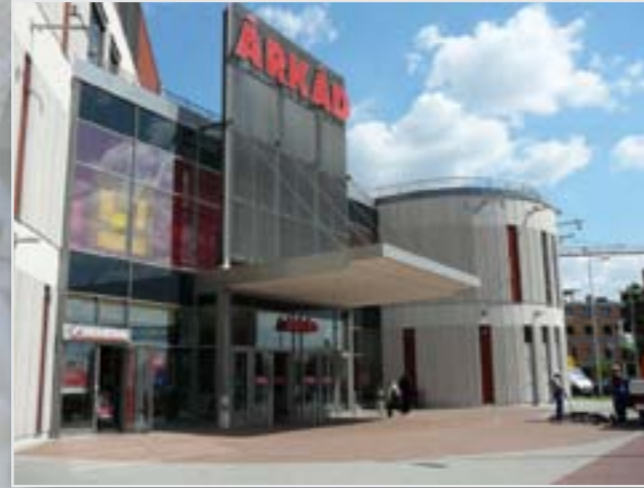
Foreroof construction of main entrance
