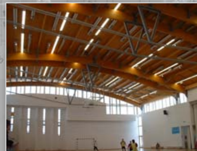
Sport Center Roof construction Mór, Hungary
