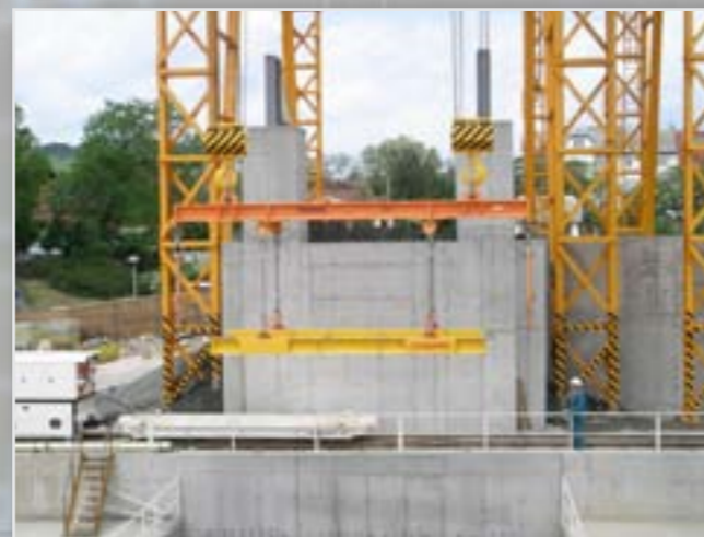
Crane lifting out from the frame
