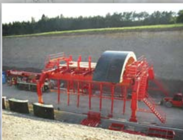
The formwork panels in assembly
