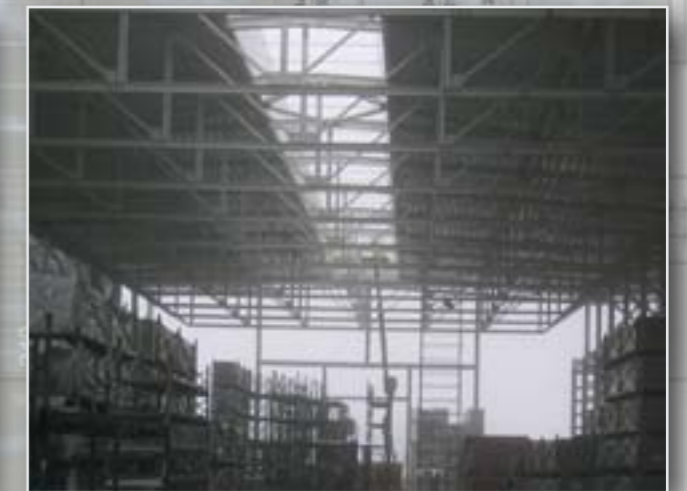
One span of the multispan structures
