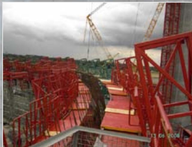
Steel platforms from the top
