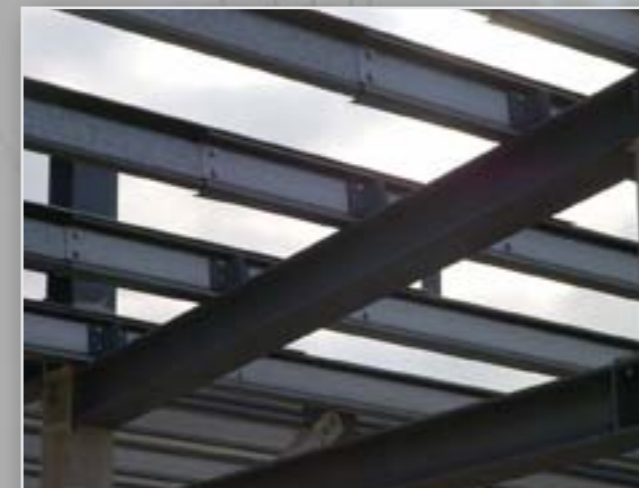
Overlapping of cold rolled profiles
