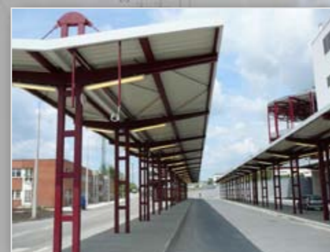
Foreroofs of bus station
