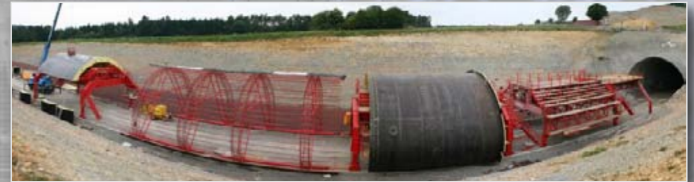
One complete, and one half complete construction next to each other
