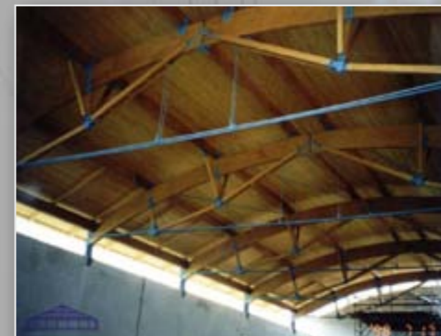
The roof structure is ready
