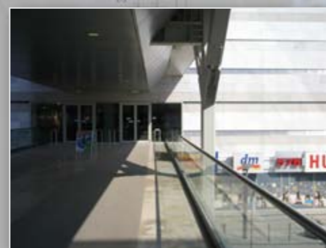
Lower level of bridge
