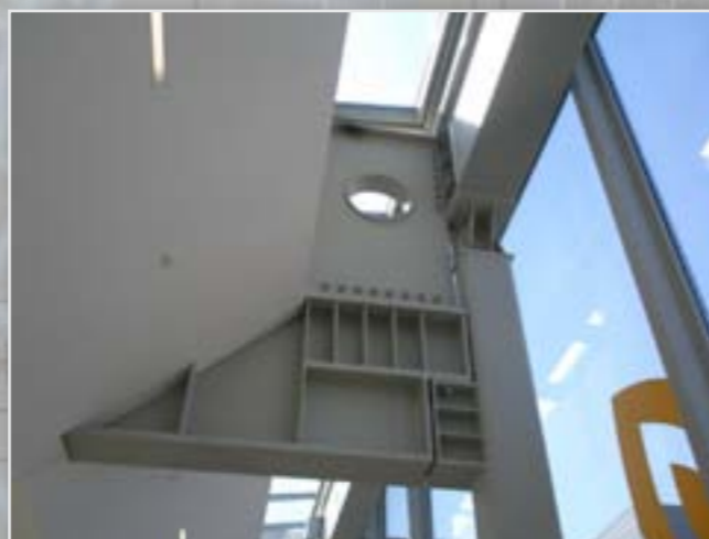
Upper part of steel bridge
