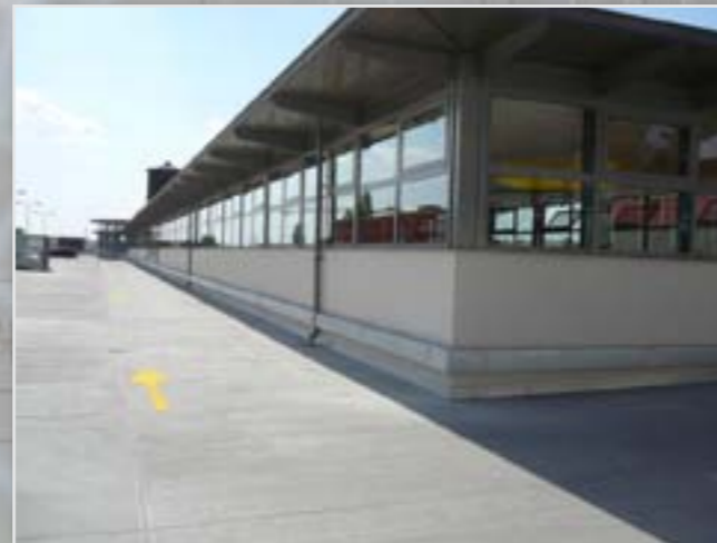
Steel beams collision protection
