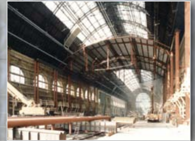
Special scaffolding at railway station
