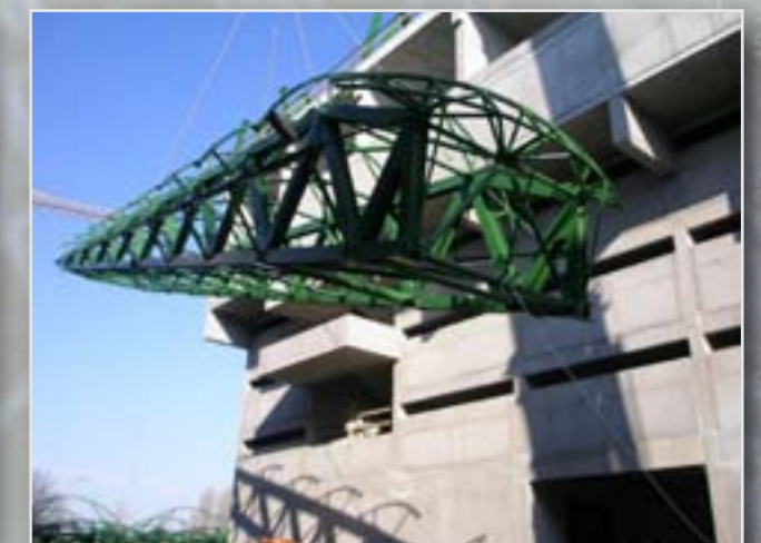
Lifting the truss beams in one piece
