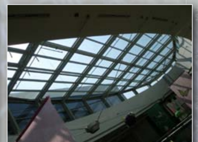
Steel construction of elliptical glass holder
