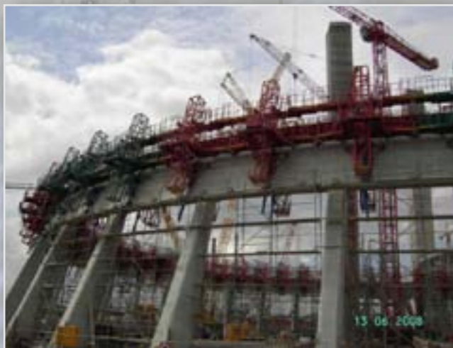
Ready to start concreting
