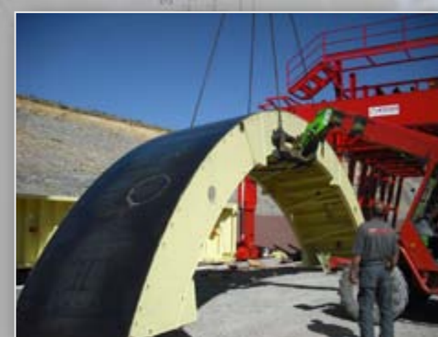
Preassembly of panels
