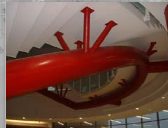
Tube construction of panoramic stair
