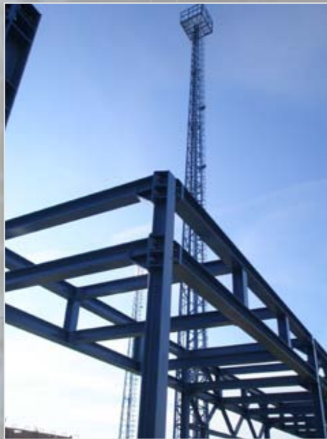
Pipe bridge with light tower
