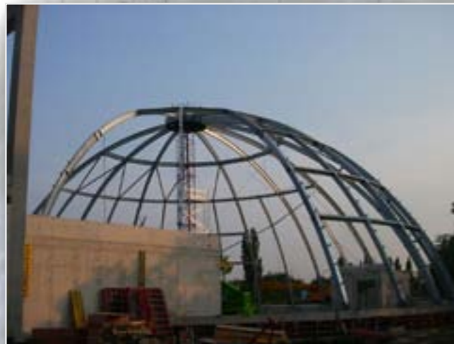
Construction beeing erected
