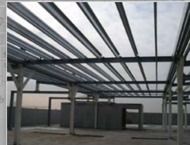
The frame construction
