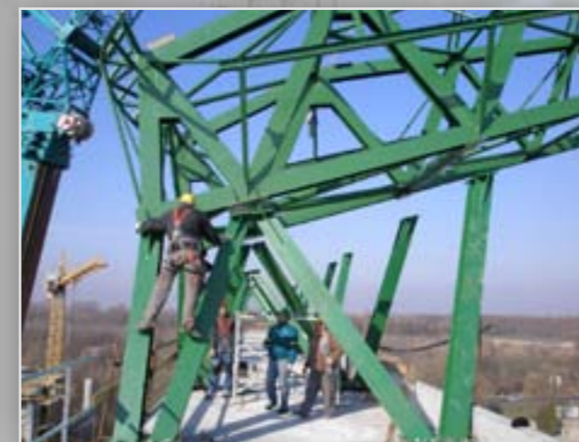
Assembling of the truss beams
