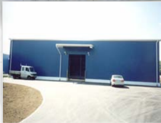
The hall with an industrial door
