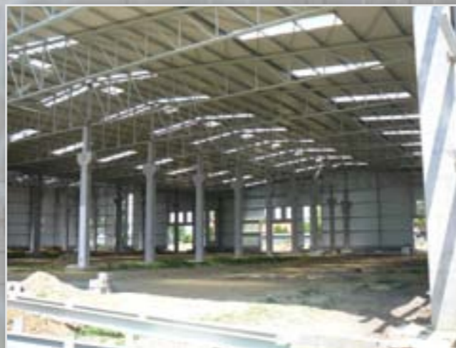
Concrete columns with steel truss-beams
